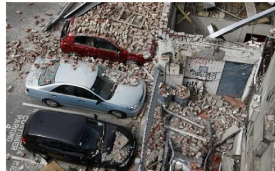
Cars lie under rubble in the central business district in Christchurch Photo: AFP/GETTY IMAGES
